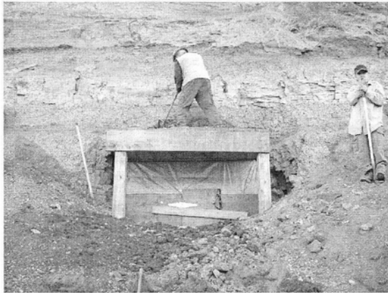
Clearing debris from the portico
